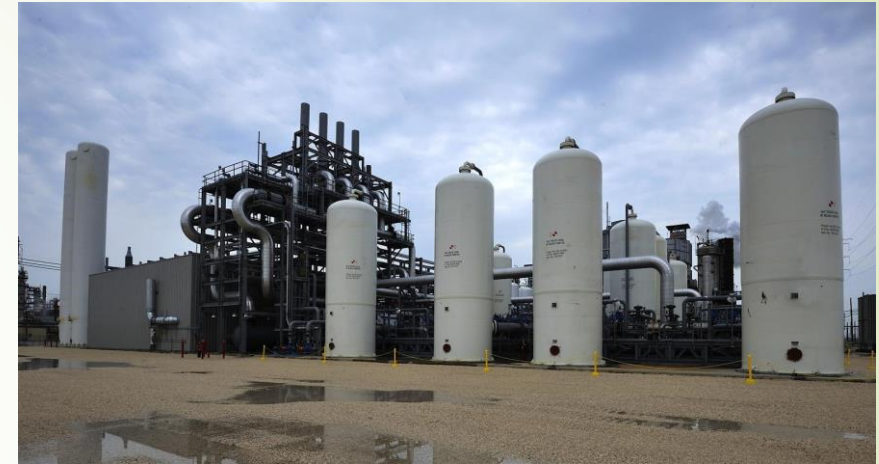
Air Products Steam Methane Reformer, Texas
