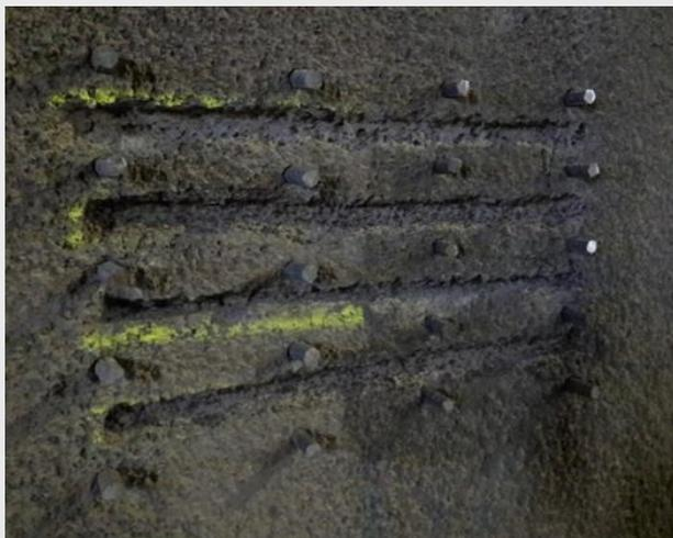
construction joint e.g. by a high-pressure water jet
