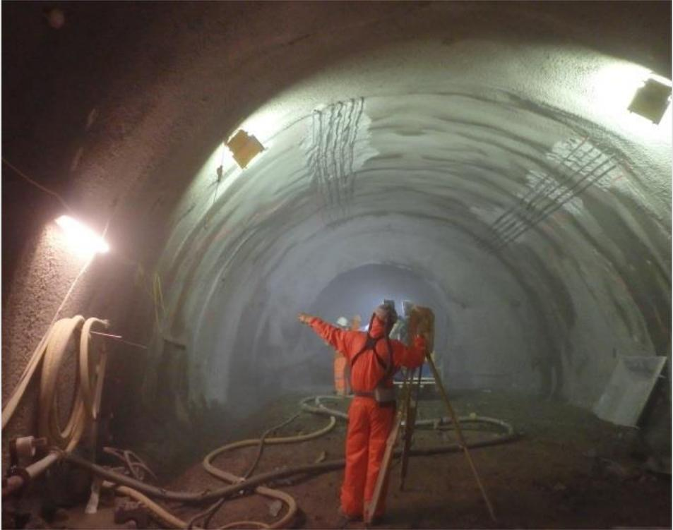
Strengthening of the shotcrete lining through a second layer, which is added subsequently
