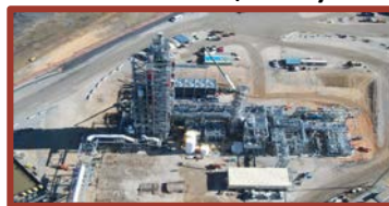
25 MW Solvent Heat Integration (Southern Company)
