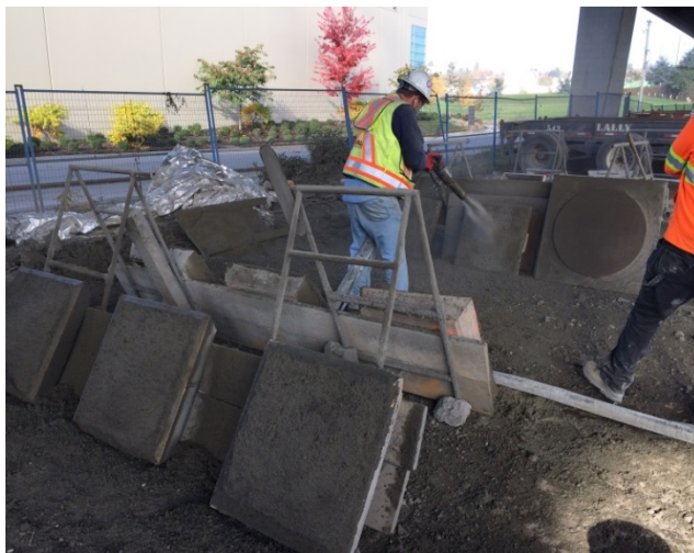
Figure 2: Shotcrete Test Panels were shot by an ACI certified shotcrete nozzleman.
