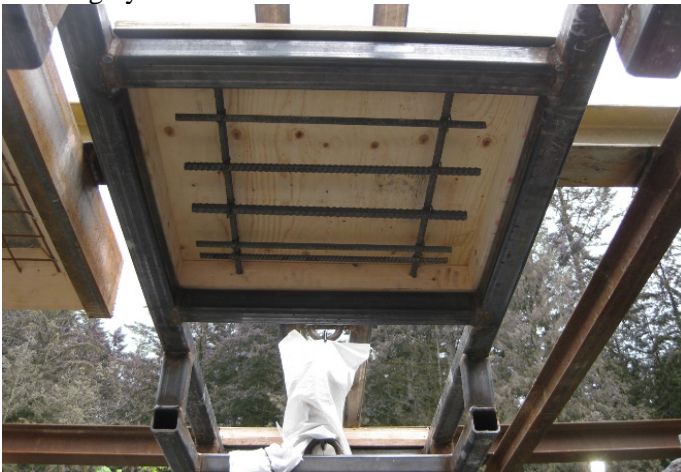
Fig. 7 ACI nozzlemans examination panel for overhead shooting
