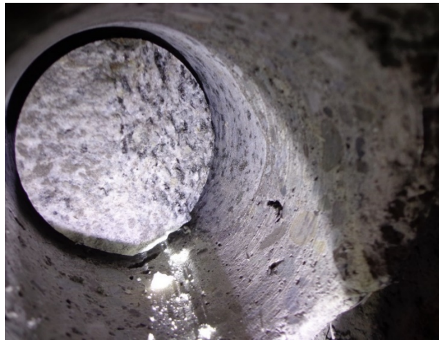
Fig. 10 Core hole from in-situ core extraction
