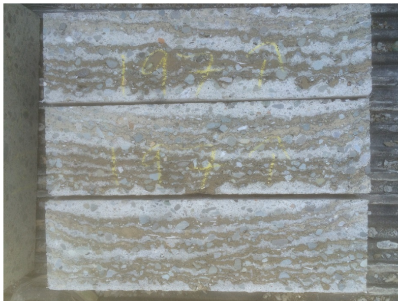
Fig.12 Defective macrosynthetic fiber reinforced wet-mix shotcrete (with accelerator) beams, layers of pockets and voids show over dosed accelerator.
