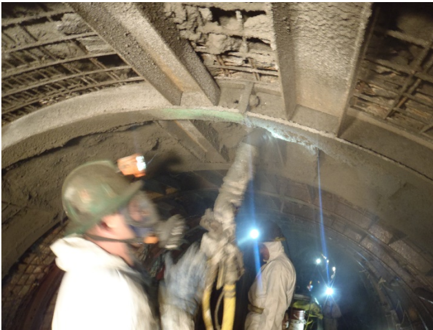
Fig. 9 In-situ mock up qualification shooting
