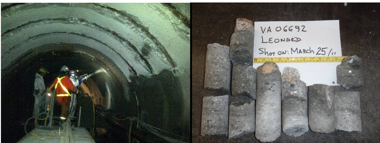
Fig. 5 Nozzleman qualification shooting with FRS for a section of lattice girder. Note that robotic sprayer shot macrosynthetic fiber reinforced wet-mix with 6% accelerator. Cores show shotcrete consolidated properly around the reinforcement.
