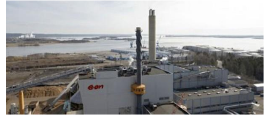
E.ON commercial waste boiler 80MWth
