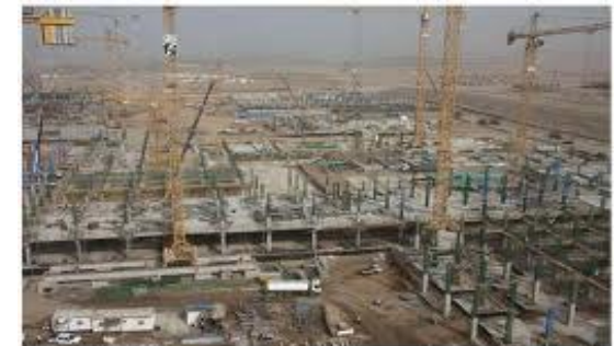
Beginning of construction in 2007
