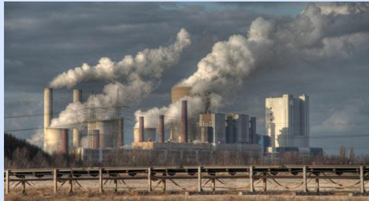
Power Plant (e.g. turbines) Industrial boilers
