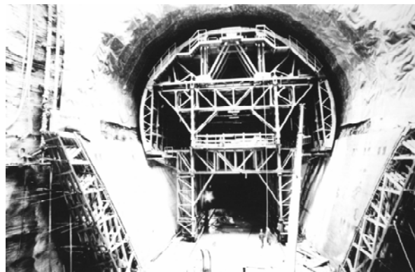
Figure 2: Waterproofing and Soffit Formwork In-Place for a Cast-in-Place Lining
