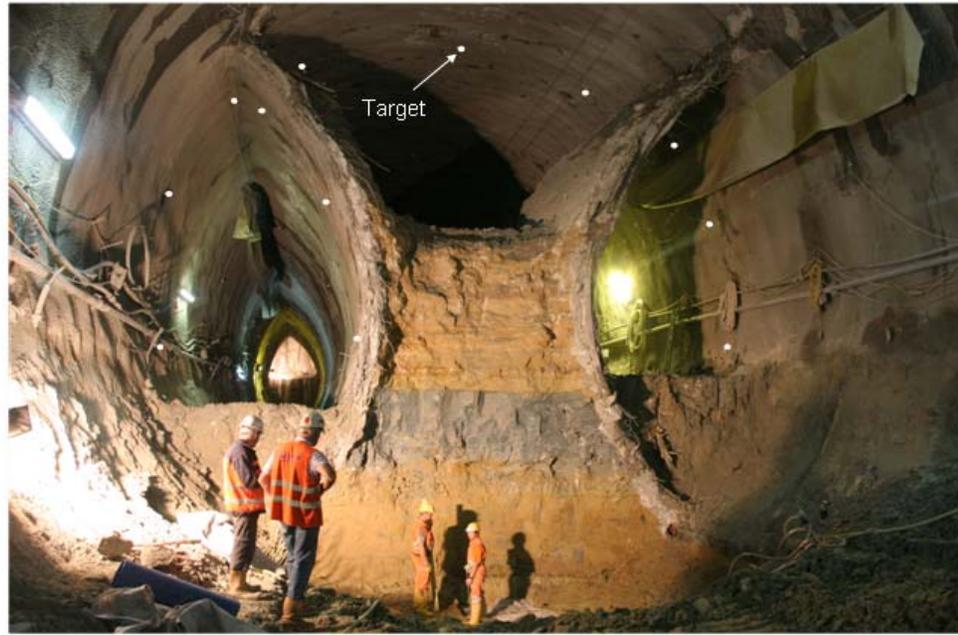
**Figure 7:** Tunnel excavated with sidewall galleries followed by core excavation (7,11); photograph showing construction works in the invert and the position of the targets.
