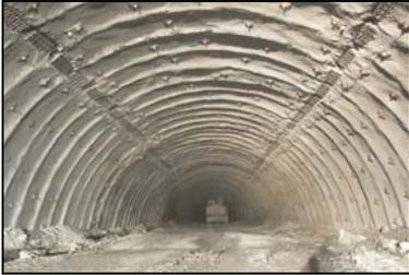
Picture 6: Support with stress controller, System Honeycomb
