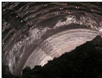
Picture 8: deformation slots
