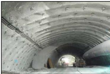
Picture 17: First use of Honeycomb in Tauerntunnel
