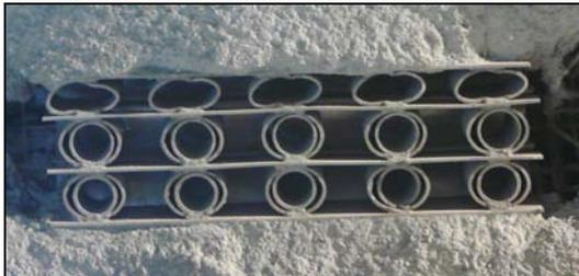
Picture 12: Honeycomb set between 2 lattice girders
