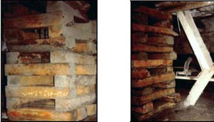
Picture 1: timber cribs
