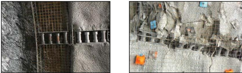
Picture 10: LSC-Elements made of deformable tube structure
