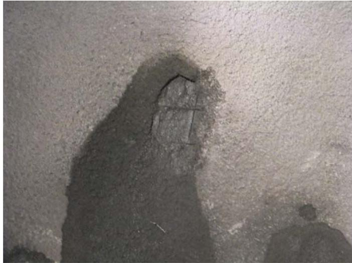
Fig. 12: Typical damage to unmodified sprayed concrete due to formation water pressure
