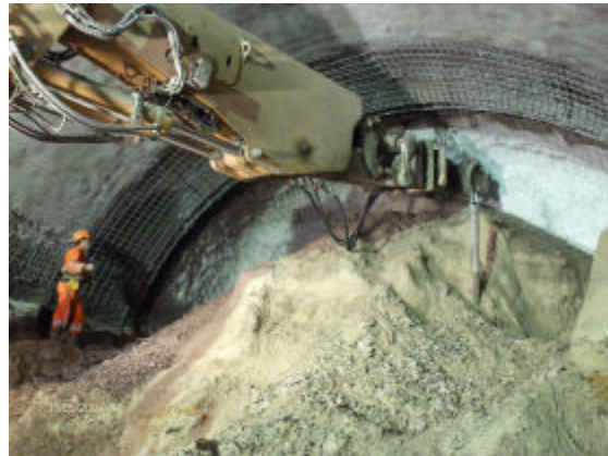
Fig. 7: Frozen ground during tunnelling
