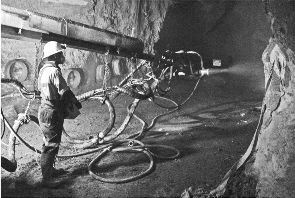
Figure 3. Spraying shotcrete over pull-out disks during in-field tests.
