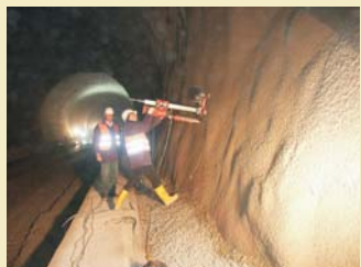
Sampling by core drilling in the Tunnel
