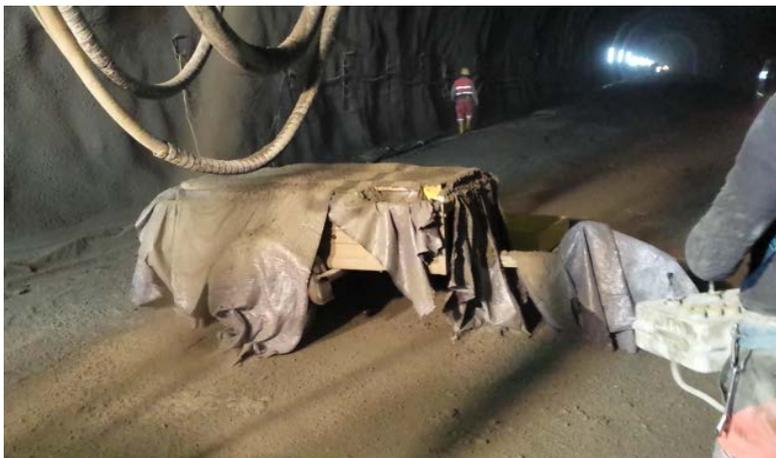
Figure 3. Shotcrete panel production on site
