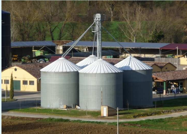
A typical reflecting painting realized on silos (Perugia, Italy)
