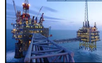
Statoil Sleipner facility: stores CO 2 in an aquifer below the North Sea
