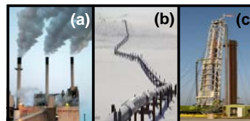
CO 2 is captured (a), transported (b) and stored (c)
