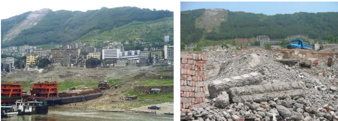
Figure 2. Yunyang, a county town, is threatened by a landslide in the rear part and to be inundated in the front part. By 2005, much of the town was demolished
