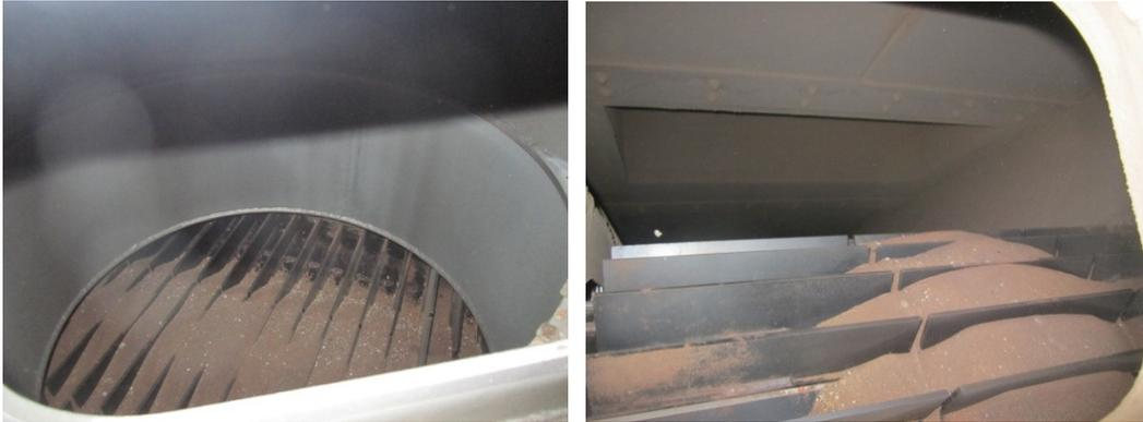
**Figure 5: Bed Ash conveyed by Superbelt®**
