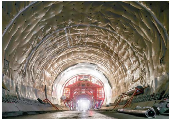
Figure 2 – Advanced self-healing and lateral flow preventing protection layer
