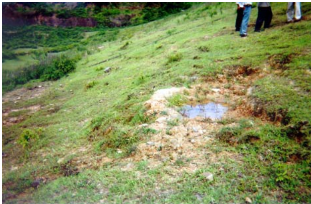
internal erosion
